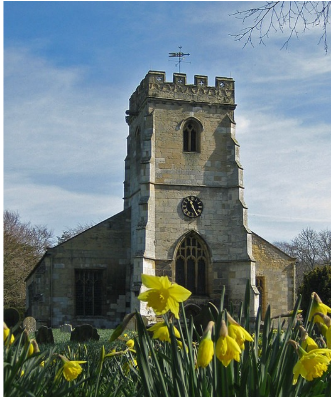
Settrington All Saints' Church
